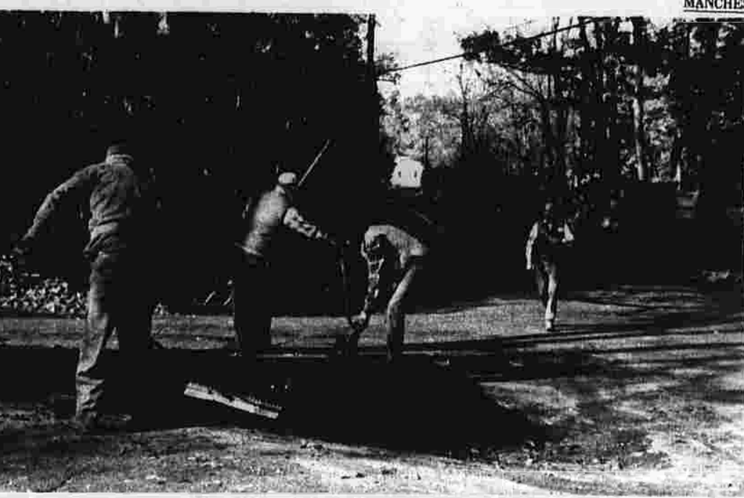
Traffic Island Removed
